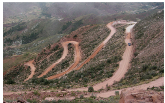
Typical road to reach the Quechua
